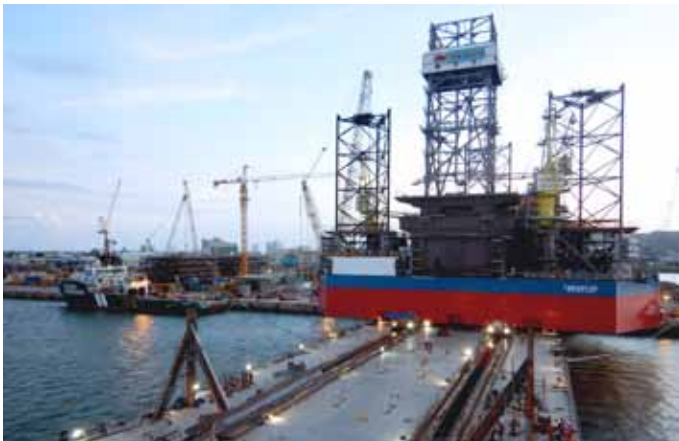
Load Out onto POSH Giant 3 by skidding operations
