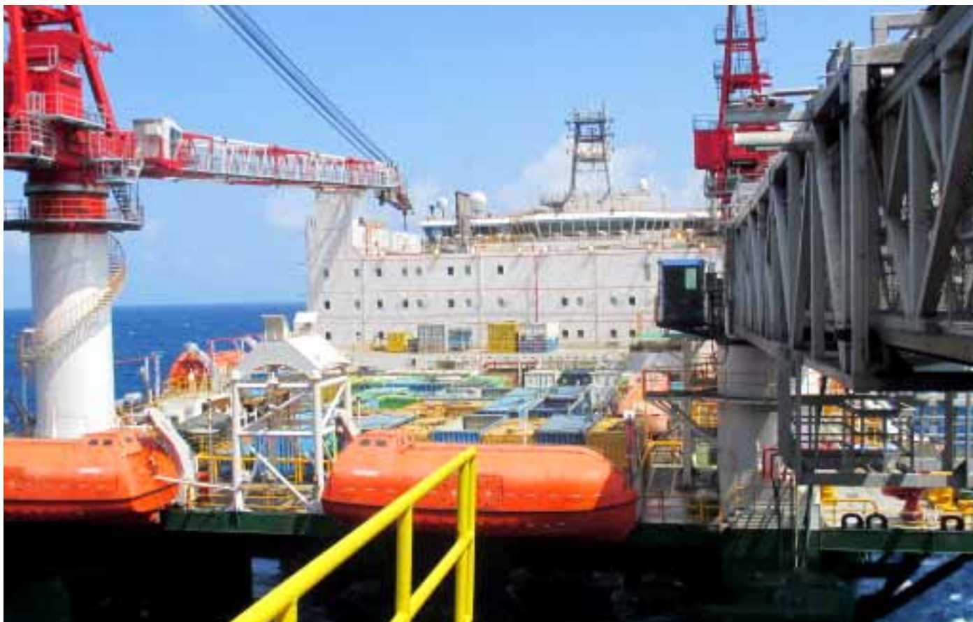
View of the large deck area on POSH Xanadu, from the FPSO platform
